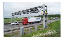
The radar and camera are mounted to a gantry leg or on an MS4 sign at the nearside of the carriageway to be enforced as shown in the pictures to the left and above.
